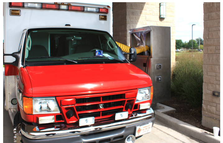
Ambulance hooked up to a MediDock, which provides power and conditioned air.
